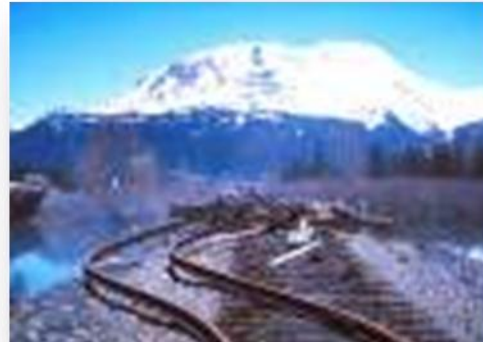
Railway line damage -Alaska
