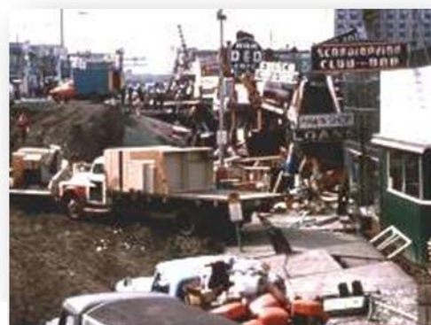
Road subsidence Shopping Centre Alaska
